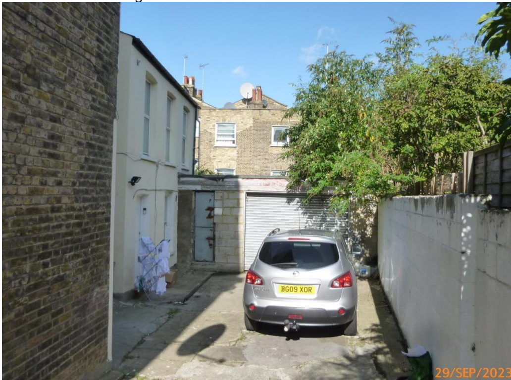
Existing garage frontage
